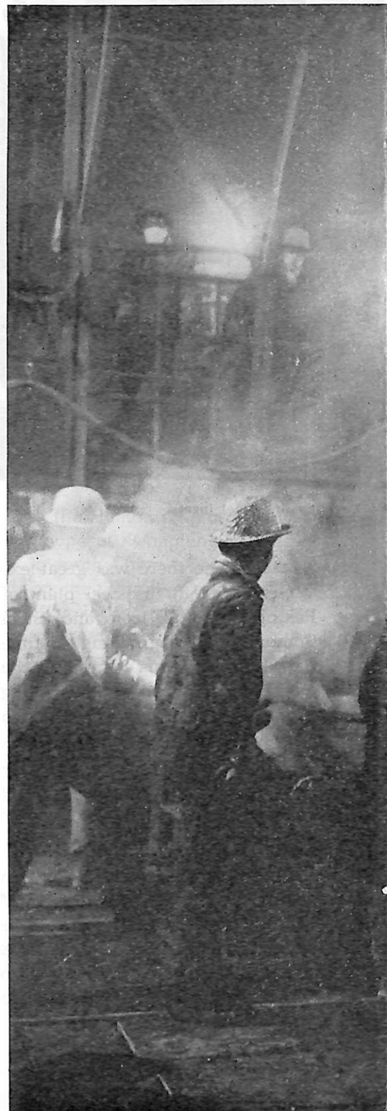
Making refractory bricks that increase the converter's life between shutdowns.
